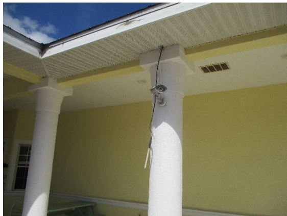
Wire hanging from soffit near front door.
