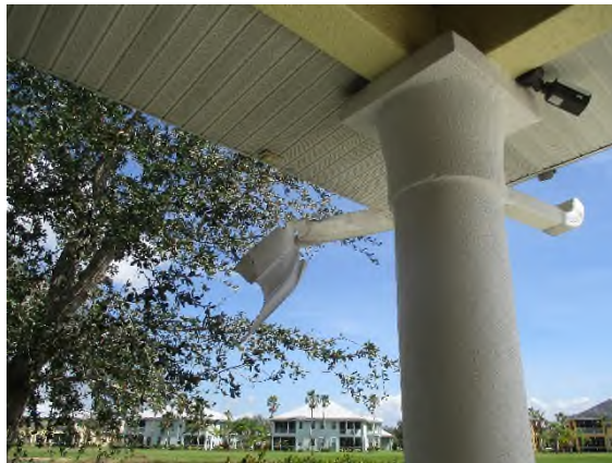
Wire hanging from soffit near front door.
