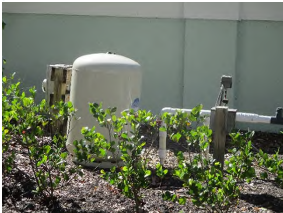
g. Pump Station #7: No issues observed.
